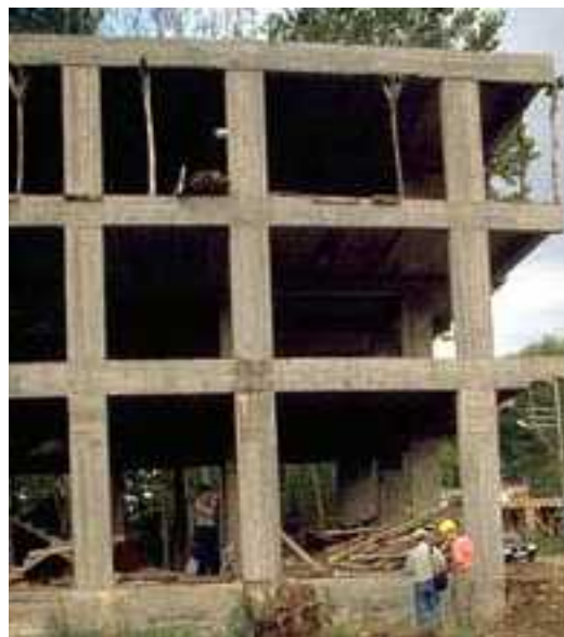
Construction of bare frame first Fig-A4
